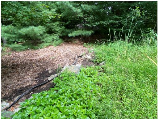
Photo 25. Plastic landscaping barrier that funnels flow from POGS1 into the upper portion of the stone swale, viewing north. (08-11-22)
