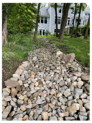
**Figure 1**. Downstream end of swale and discharge by improved stone wall end (top left); stone swale looking upstream, photo taken from area close to stone wall end (right); property directly north of swale subject to erosion, looking upstream, photo taken from area close to stone wall end (lower left).
